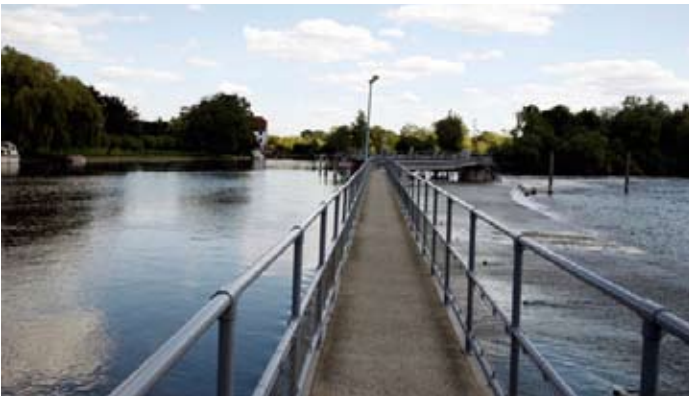
Hambledon Weir, UK
