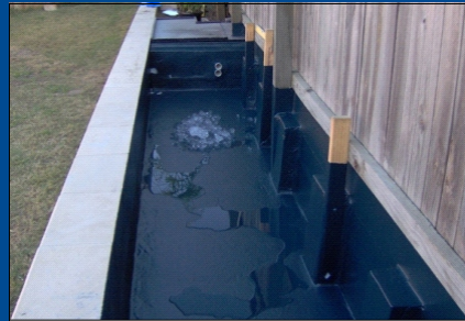
Water feature - ready to fill within the hour
