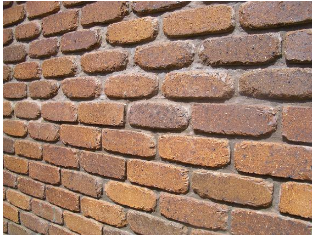
close up of bricks
