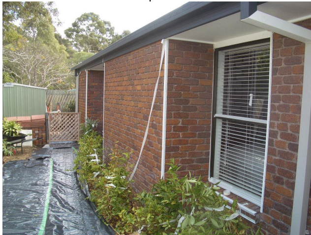
preparation of bricks
