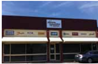
Adelaide Automation & Control
