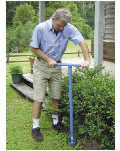
Using auger to place Exterra Station.
