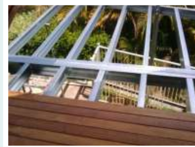
Beginning of job
