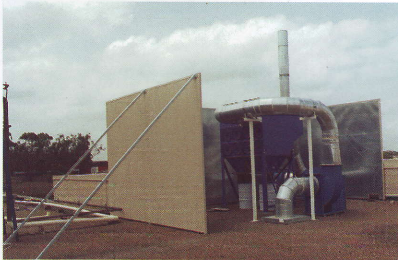
ACOUSTIC SHIELDING FOR DUST COLLECTION SYSTEM FOR MERCK SHARP AND DOHME
