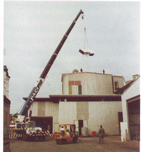
SITE INSTALLATION OF FAN DISCHARGE SILENCER
