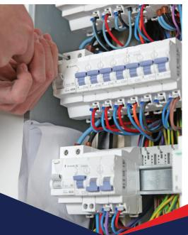
Safety switches can corrode, especially in coastal areas. This prevents them from operating correctly when they need to prevent a fatal shock.
