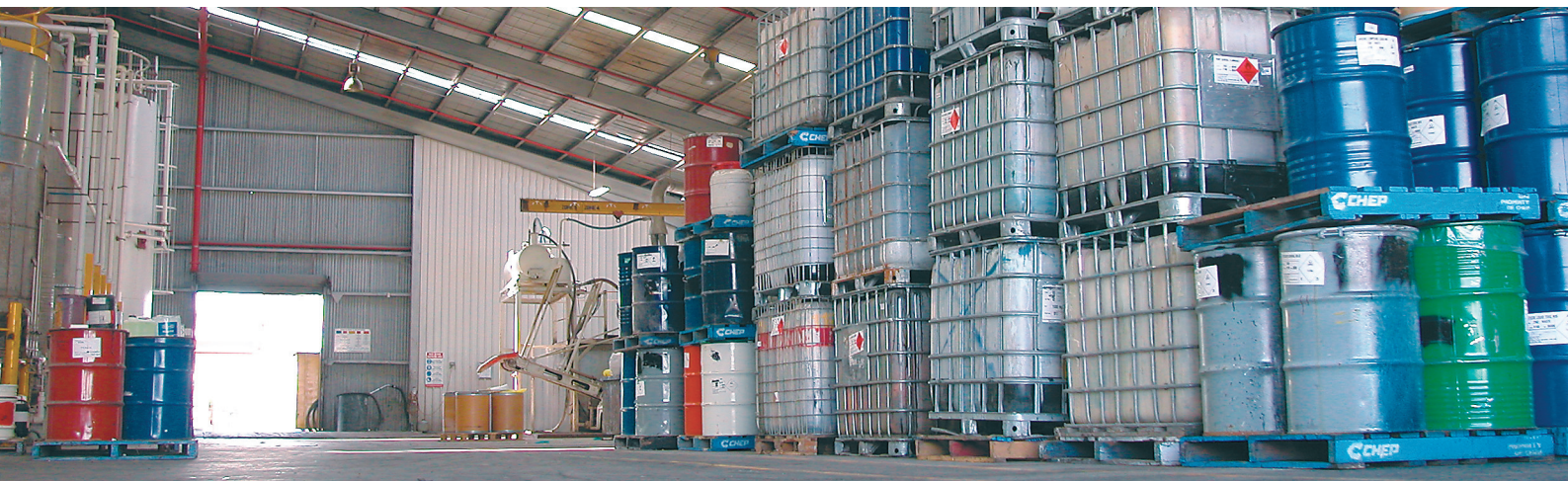
Above: Treatment and storage facilities. Cover: Hazpak3000 Densification System
