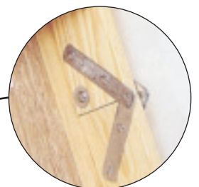
Metal hinges riveted on both sides of rail joints prevent side to side movement
