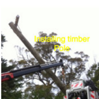
Installing timber Pole
