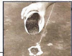
Rebuilding Damaged Floors
