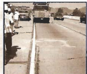
Rebuilding Damaged Freeways
