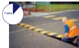
Put modules in place
