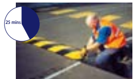
Trim rubber & clean site
