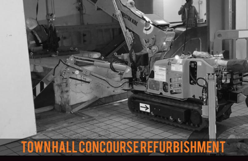
Perfect Contracting were engaged to complete detailed demolition, including removal of tile and bedding, concrete cutting and grinding, as part of Sydney Trains major renovation of Town Hall Train Station. The works involved precise operation of demolition tools, including Hilti jackhammers, Hilti wall grinders, Hilti floor grinders, oxy cutting equipment, along with various other specialised equipment. The project consisted of the removal of the structural floor above the escalators.
