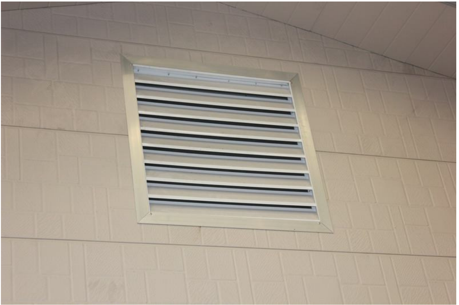
Aluminium Shutter Window: 800 x 600mm.
