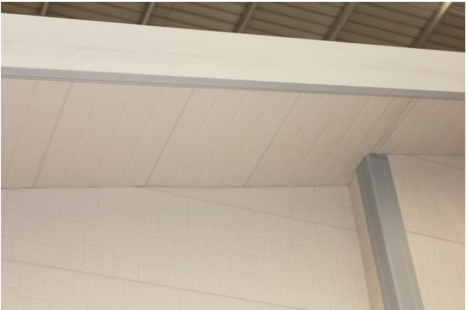
Eave ceiling plate is different using wall decoration plate.
