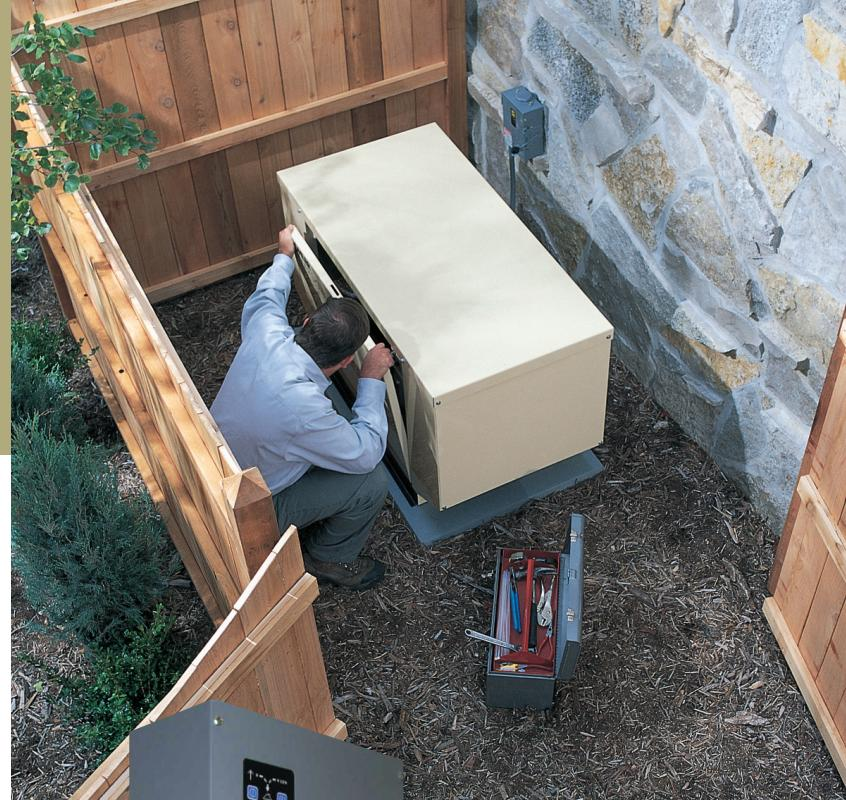
Slightly larger than the main distribution panel, the automatic transfer switch is mounted inside or outside your home and exercises the generator regularly so it's ready when you need it most.
