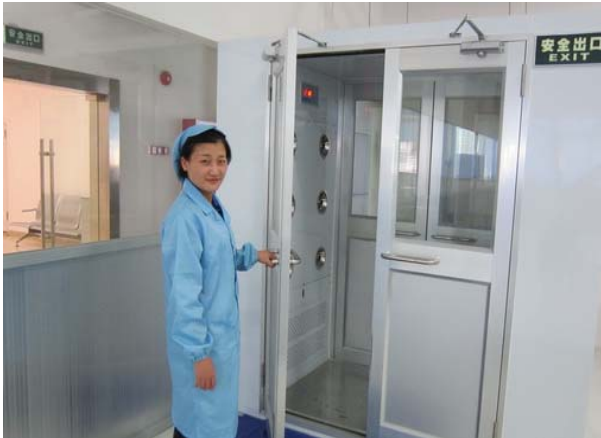
Air Shower Entry Chamber for Workshop
