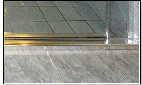
Bottom detail of a front-only screen, showing aluminium channel and polycarbonate strike along bottom of door, protecting against leakage
