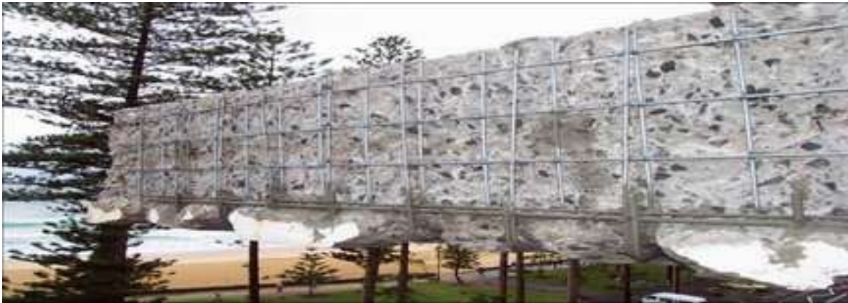
Surfways, Manly Spalling concrete and facade upgrade
