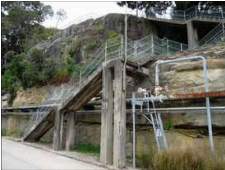
Heritage Structures, Cockatoo Island Spalling Concrete
