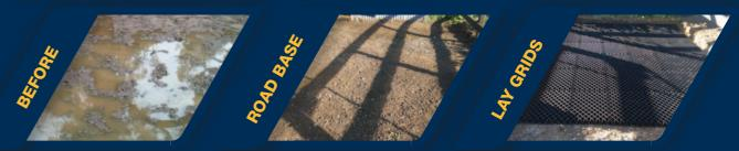
ROAD BASE - Lay 50mm of road base to give a solid, level surface to lay the grids on.
