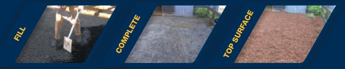
FILL - Fill the grids with 10mm gravel to assist drainage. TOP SURFACE - Sand, wood shavings & wood chip are popular choices for surfaces in day yards.
