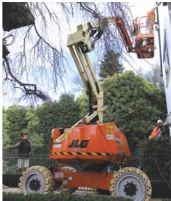
The boom lift provided a work platform height of 34ft (10.31m).
