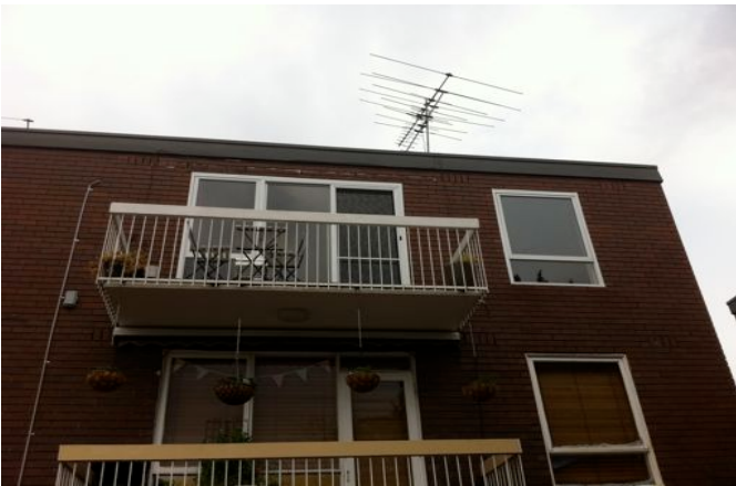
Aluminium Sliding door and Awning Window- top floor replacement Rosebud
