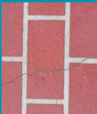
Cracking
