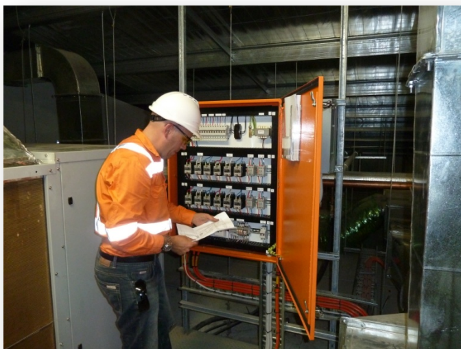
The testing & inspecting of our sub-contractors works is critical.
