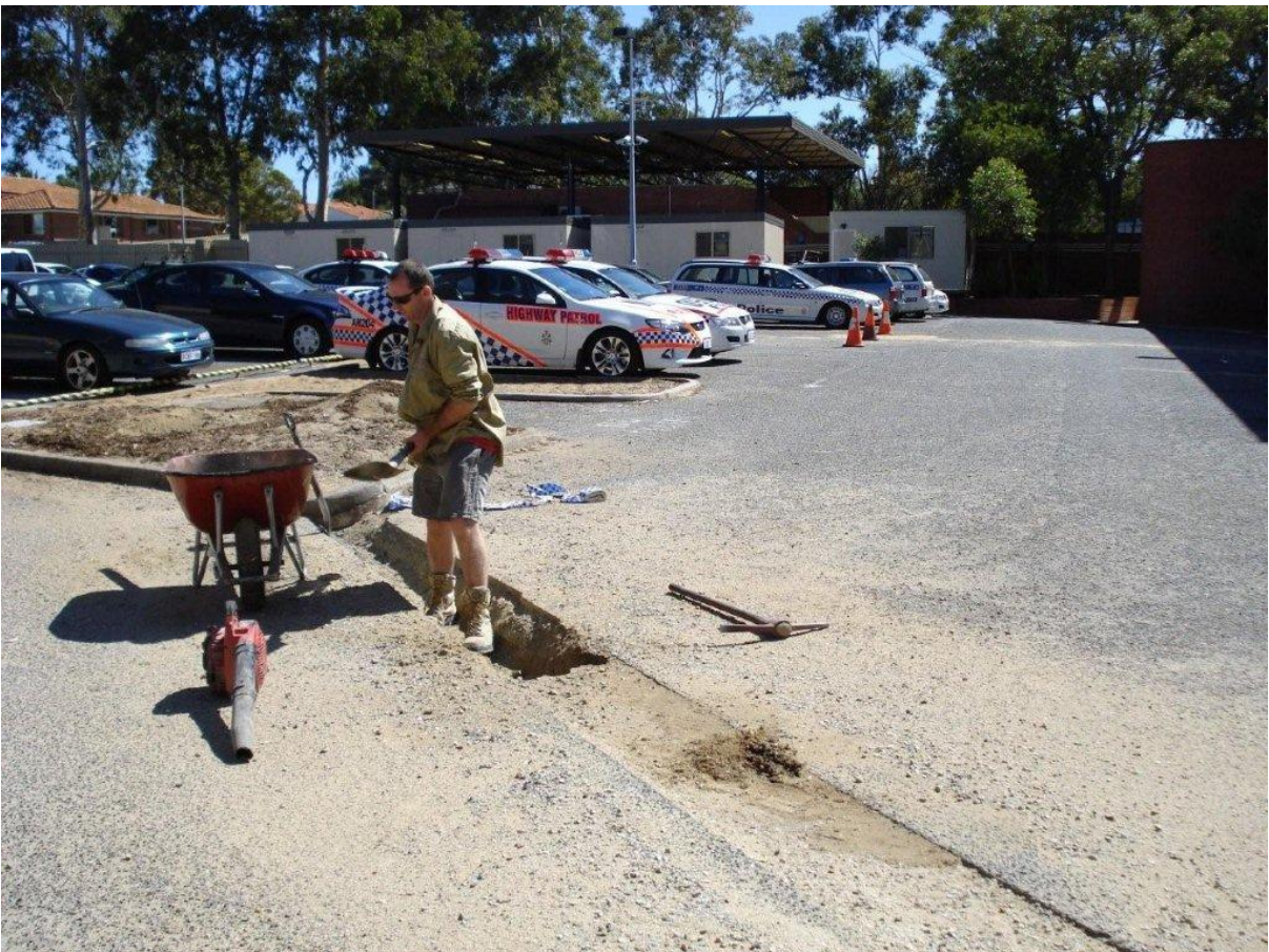
Figure 4 Warwick Police Station - Trench Reinstatement
