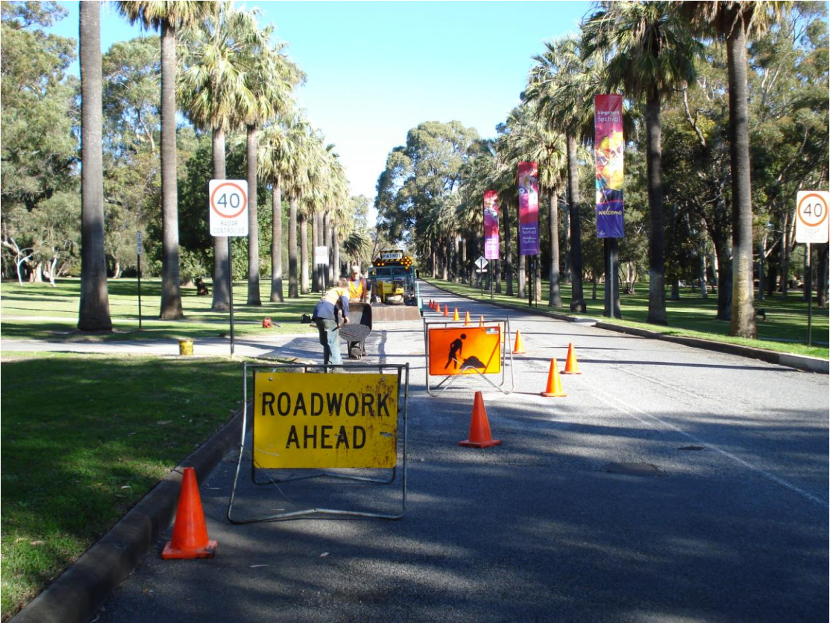
Figure 1 Kings Park & Botanic Garden - Section Repairs
