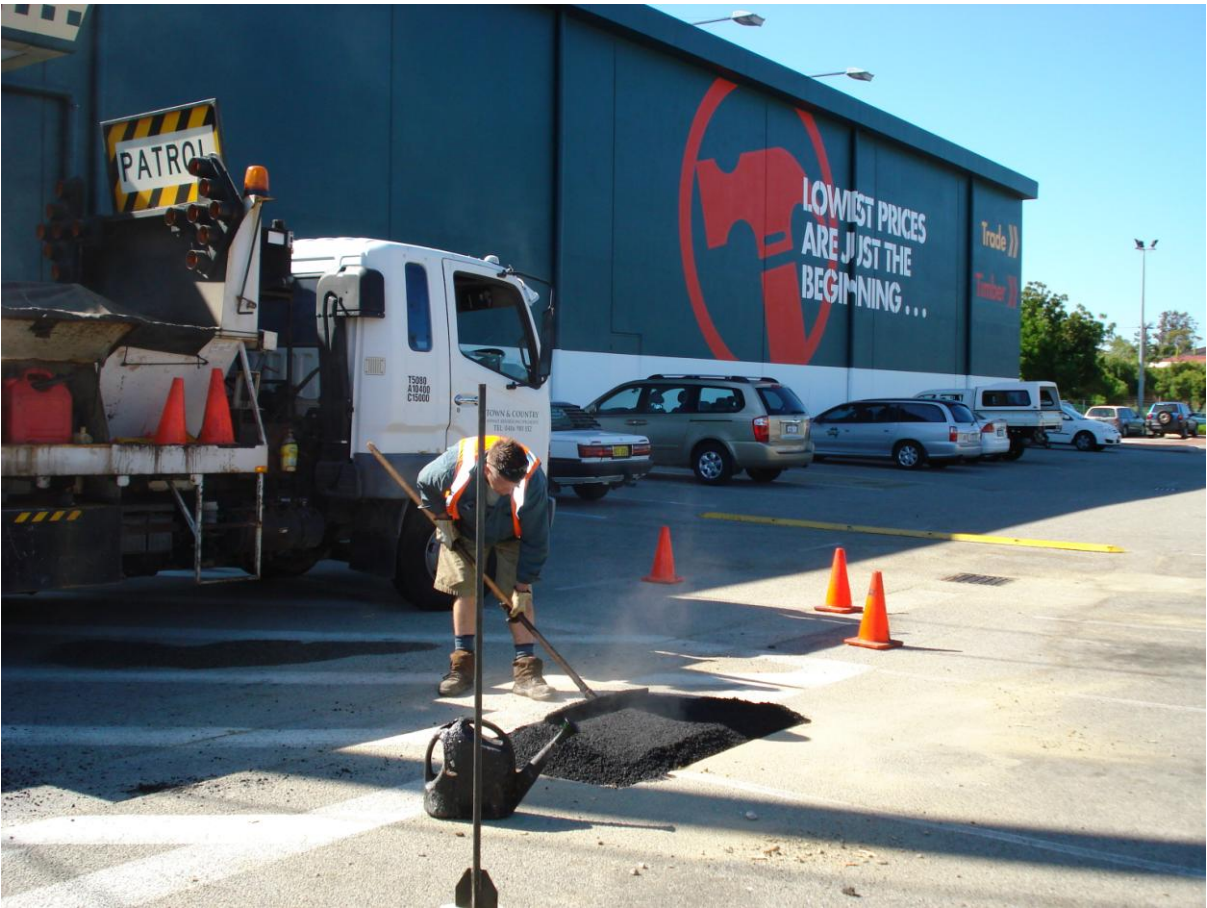
Figure 3 Bunnings Warehouse - Section Reinstatement
