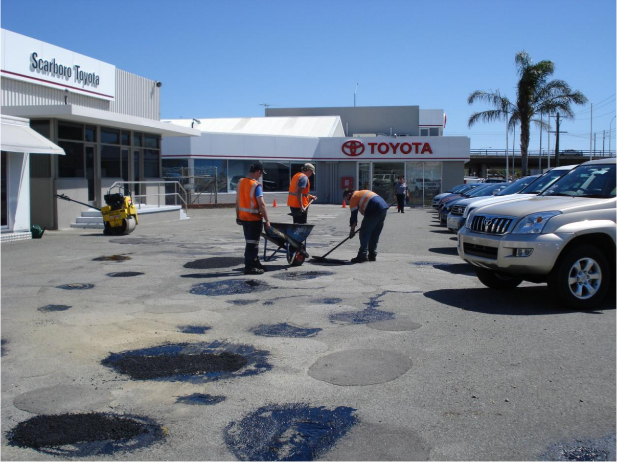
Figure 2 Scarboro Toyota - Pothole Repairs
