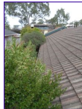
i suggest these trees be trimmed back to prevent the gutters blocking up from falling leaves, this will also help prevent pests such as possums having easy access to your roof void.
