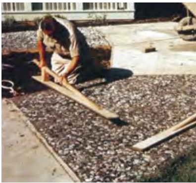
Figure 25 The aggregate is initially tamped with wood floats or screeding boards.
