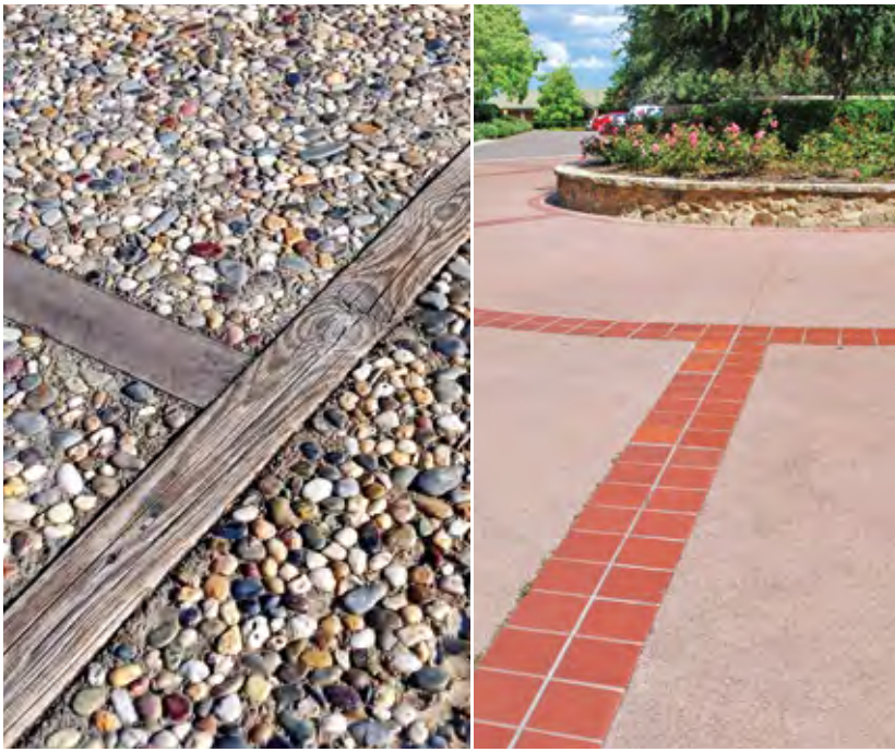
Figure 50 Use of various materials to form/conceal joints
