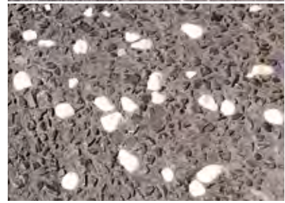
Figure 17 Surface seeded with large decorative white quartz aggregate (Mt Keira Summit Park, NSW)
