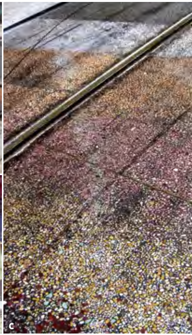
Figure 16 Decorative aggregate used as feature in Bourke Street Mall, Melbourne (Artist: David Humphries, Public Art Squad) [a] Seeding aggregates onto surface [b] Floating aggregates into surface [c] Surface after honing
