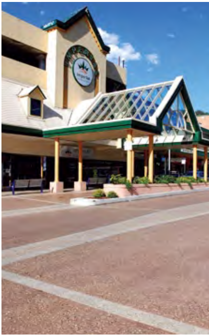
Figure 13 Matrix coloured to complement the aggregate colour and to differentiate areas of pavement
