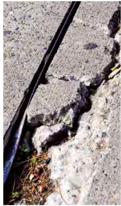
Figure 46 All movement joints should be sealed to prevent ingress of debris causing spalling of edges
