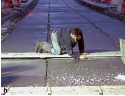
Figure 16 Decorative aggregate used as feature in Bourke Street Mall, Melbourne (Artist: David Humphries, Public Art Squad) [a] Seeding aggregates onto surface [b] Floating aggregates into surface [c] Surface after honing
