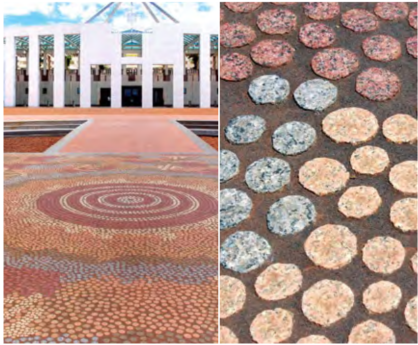
Figure 19 Polished stone (aggregate) embedded in cement mortar topping (Mural in forecourt Parliament House, Canberra)
