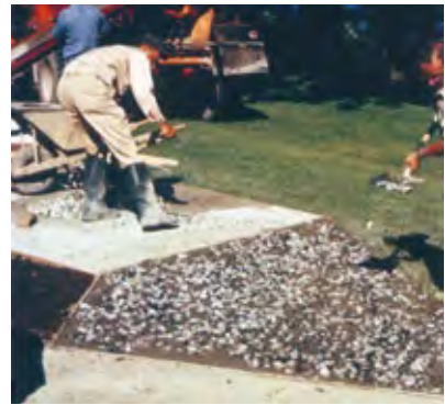
Figure 24 Selected aggregate is sprinkled evenly over the surface. In this example a combination of black and white crushed stone is used
