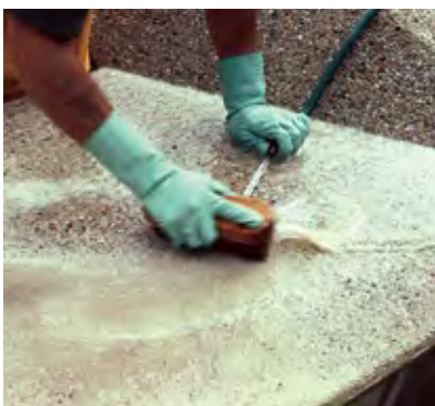
Figure 28 Hand washing of smaller areas may be more practical than using a broom
