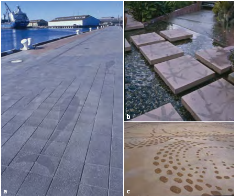
Figure 33 Patterns/pictures can be formed by either masking the object [a] and abrading the surrounding surface or masking the surrounding area [b] and [c] and abrasive blasting the actual object/pattern
