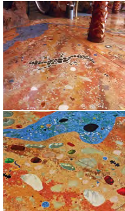
Figure 12 Glass aggregates provide a translucent feature in artistic terrazzo design (Star City Casino, Sydney)
