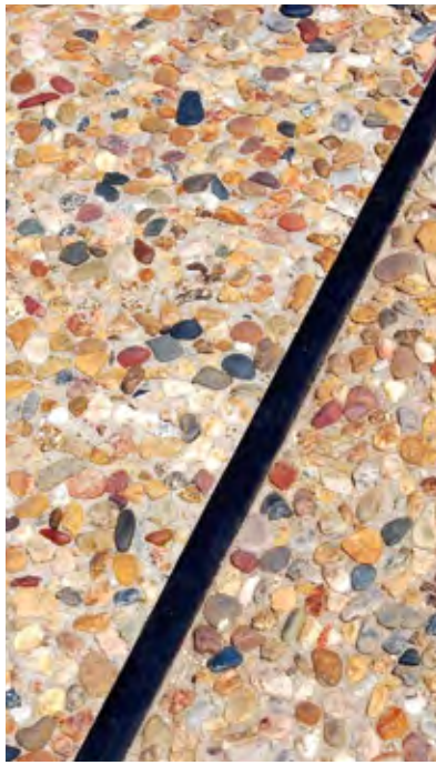
Figure 45 If gaps open along edges of pre-formed strips, the joint should be sealed to prevent ingress of debris
