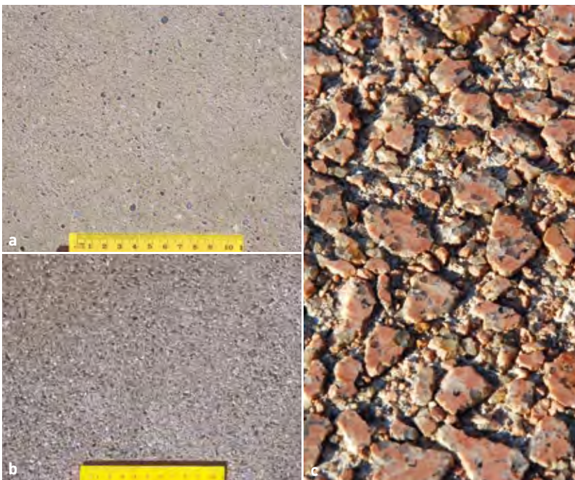
Figure 40 Levels of acid etching [a] Light acid etch with fine aggregate and some coarse aggregate exposed [b] Medium acid etch with top of coarse aggregate exposed [c] Heavy acid etch exposing honed top of coarse aggregate
