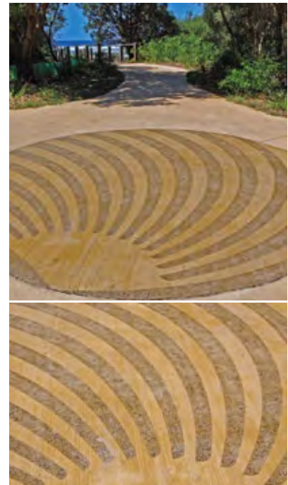
Figure 34 Shell pattern formed by abrasive blasting over a specially cut rubber-back-vinyl stencil
