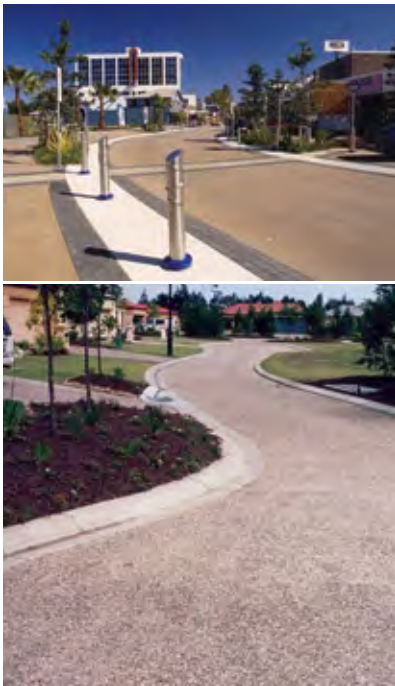
Figure 10 Exposed aggregate surfaces for local roads and residential streets
