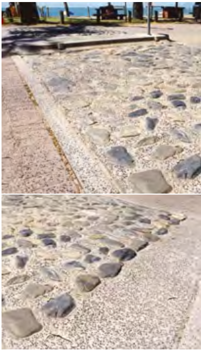
Figure 4 Large stones ('plumbs') set into concrete surface as traffic-control device
