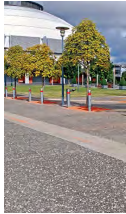
Figure 6 20-mm basalt and white quartz aggregates used for roadway
