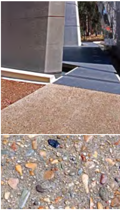
Figure 7 Exposed aggregates of 'normal' concrete mix
