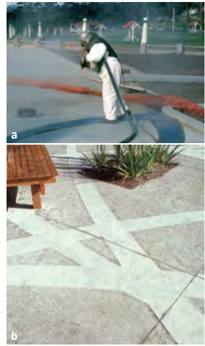
Figure 31 Abrasive blasting surface [a] and end result [b] . Stencils consisted of specially cut thin steel plates
