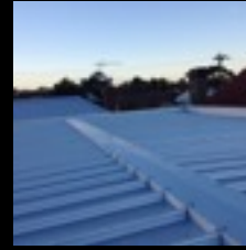
Northcote Zinalume KlipLok Roof
