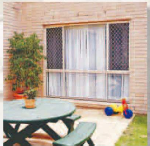
Window grilles to sliding sashes only
