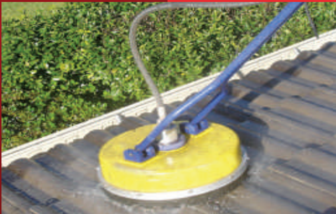
Cleaning of Roof Surface
