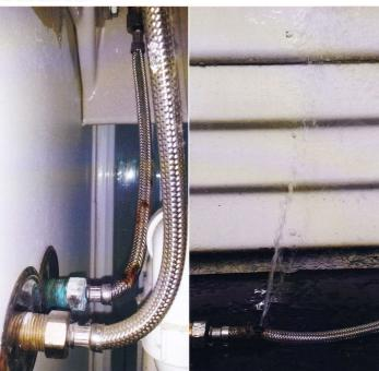
This image shows a burst hose which can happen at any time to a rusty or damaged hose and cause extensive damage from flooding in the home.
