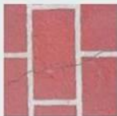
Cracking
