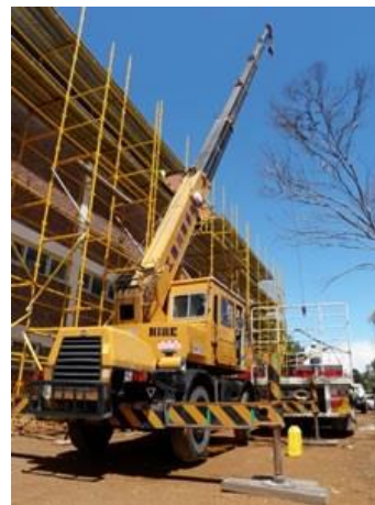
Typical single pole putlog scaffold
