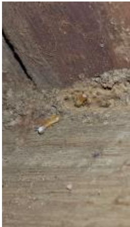
Live Termite to Bearer and Mudding to Joist
